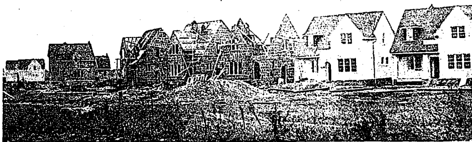
LANSLOWNE PARK ESTATE, BRANTFORD, ONT., SHOWING TYPE OF HOUSES BEING ERECTED FOR THE DOMINION STEEL PRODUCTS COMPANY. SCOTT & WARDELL, ARCHITECTS.
