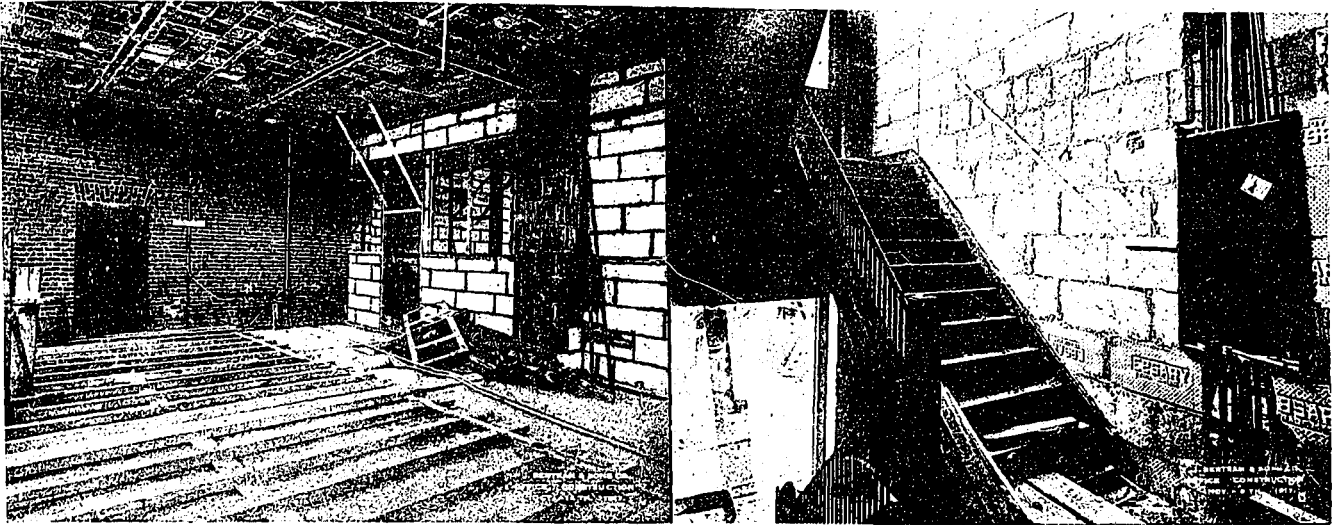
PROGRESS VIEW SHOWING GYPSUM BLOCK PARTITIONS AND HOLLOW TILE FLOORS WITH CINDER FILL AND NAILING STRIPS FOR HARDWOOD FINISH. OFFICE BUILDING OF JOHN BERTRAM & SONS COMPANY, DUNDAS, ONT.
