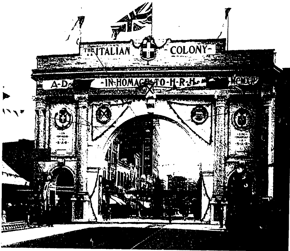
THE ITALIAN ARCH—THIS GRACEFUL ARCH WAS ERECTED IN HASTINGS STREET BY THE ITALIAN COLONY
