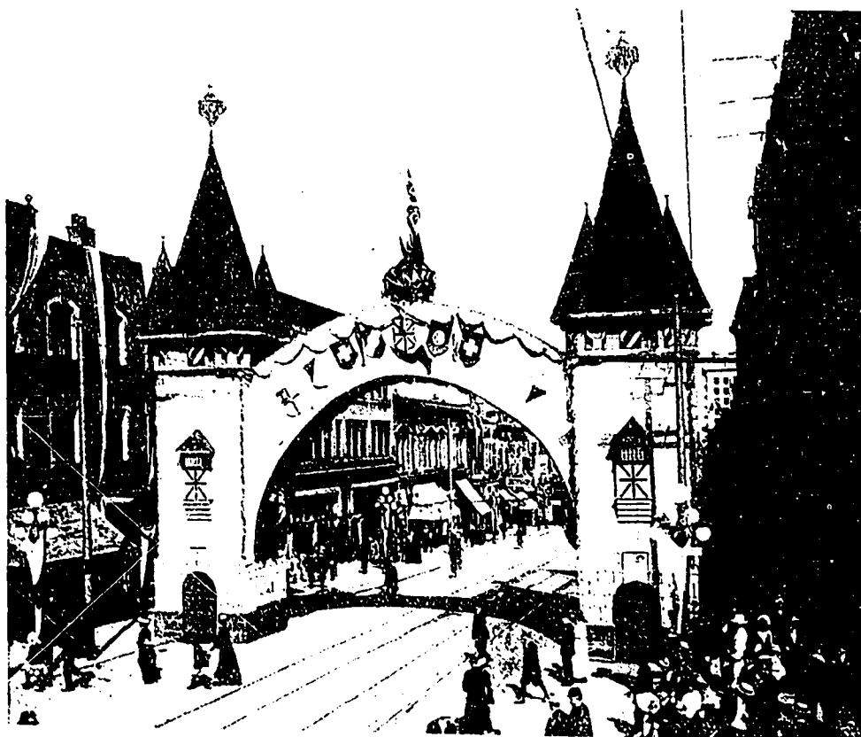
THE GERMAN ARCH—THIS ARCH, ERECTED IN GRANVILLE STREET, CLOSE TO THE VANCOUVER HOTEL, WHERE THE ROYAL VISITORS STAYED, WAS A REPRESENTATION OF A GATEWAY OF A MEDIEVAL GERMAN TOWN
