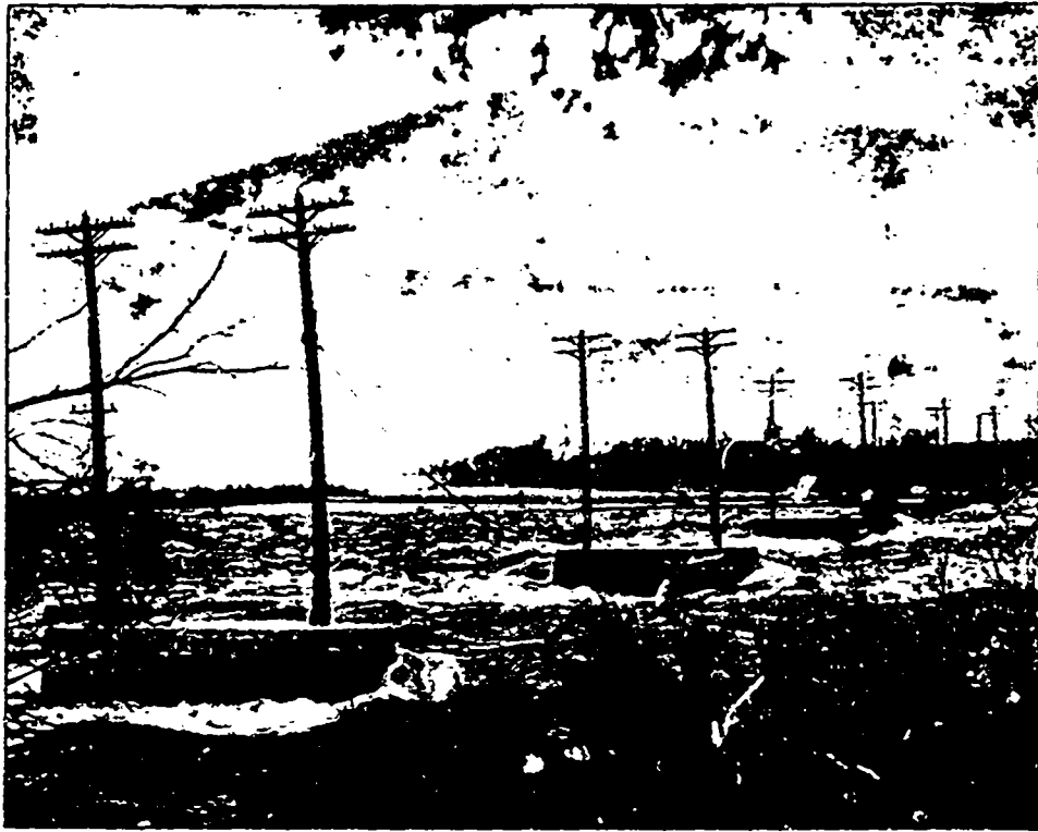
DOUBLE POLE LINE CROSSING THE RIVER AT CHAMBLY.
