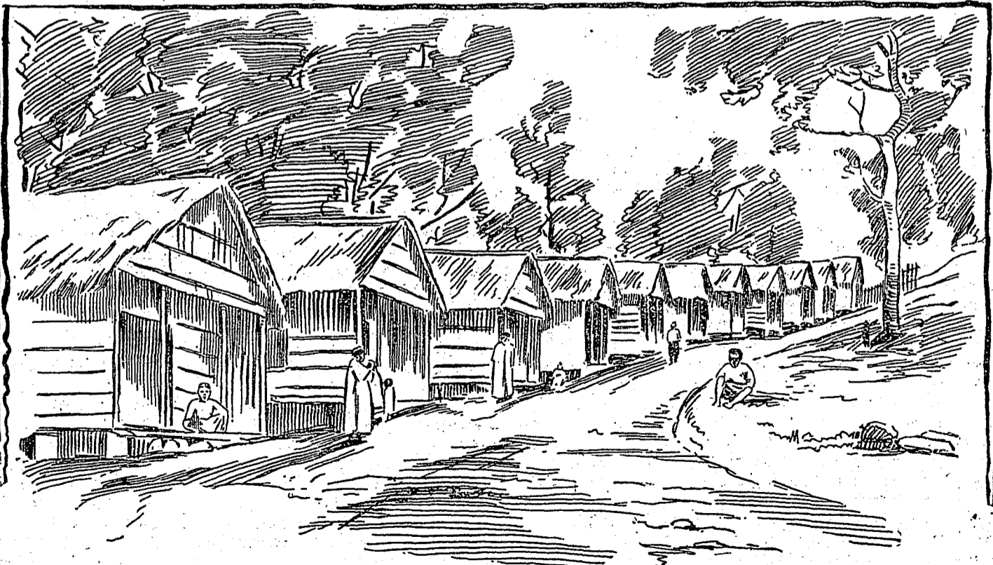
AND NOW—STUDENTS' HOUSES, VATORATA.
