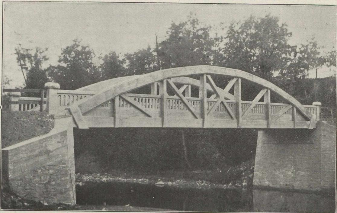
A Concrete Truss Bridge on the Middle Road, between the Counties of York and Peel, Ont.
