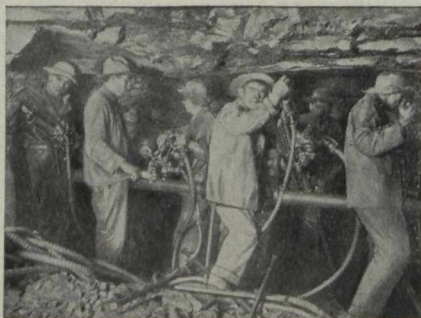
Sullivan Liteweight Water Drills in the Mt. Royal Tunnel, Montreal
