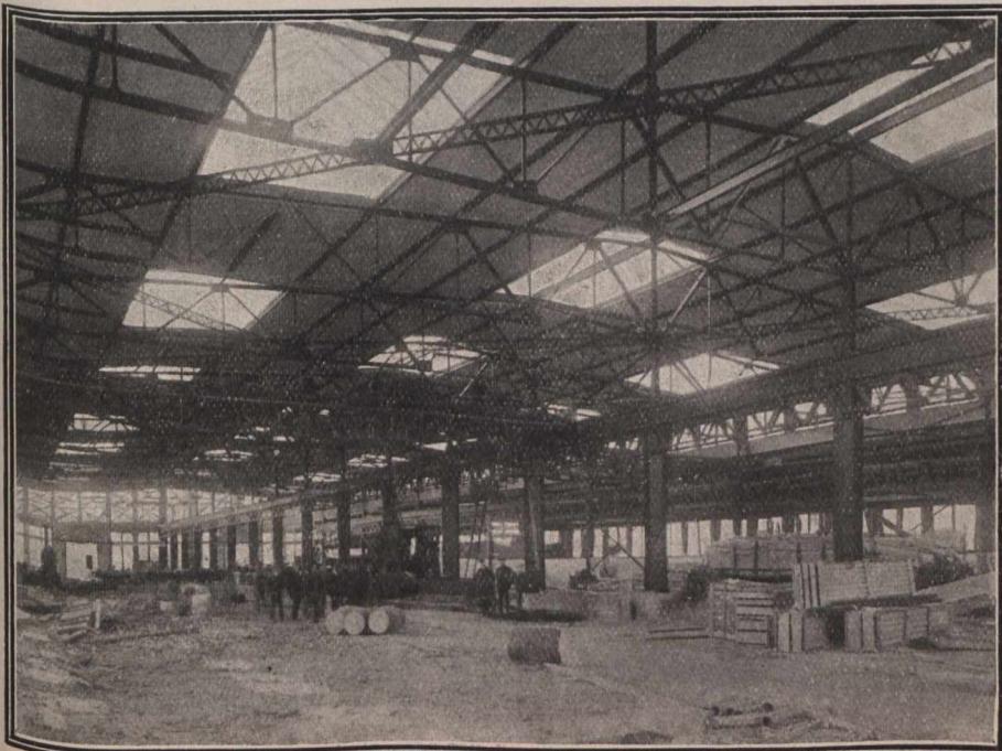
INTERIOR OF MACHINE SHOP, INTERCOLONIAL RAILWAY, MONCTON.
