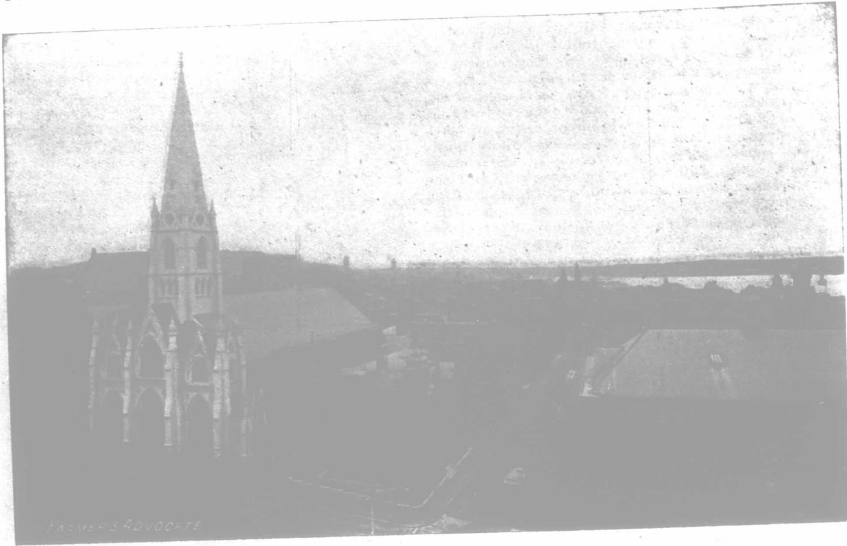
BARRINGTON STREET, HALIFAX—LOOKING NORTH.
