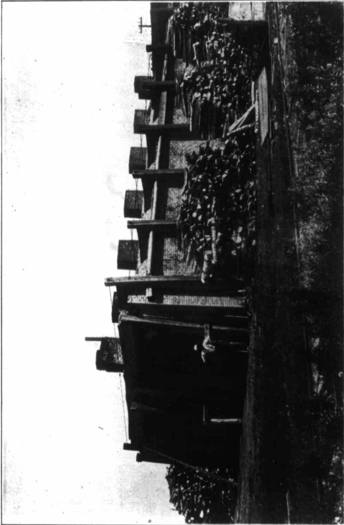
UP AND DOWN DRAFT RECTANGULAR KILN USED AT STEPHEN'S BRICK YARD, PORTAGE LA PRAIRIE, FOR BURNING BRICKS, MADE BY SOFT MUD PROCESS.
