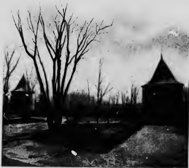
Towers in the Grounds of Montreal College, Sherbrooke Street. probably the Oldest Structure in Montreal, dating back some 250 years.
