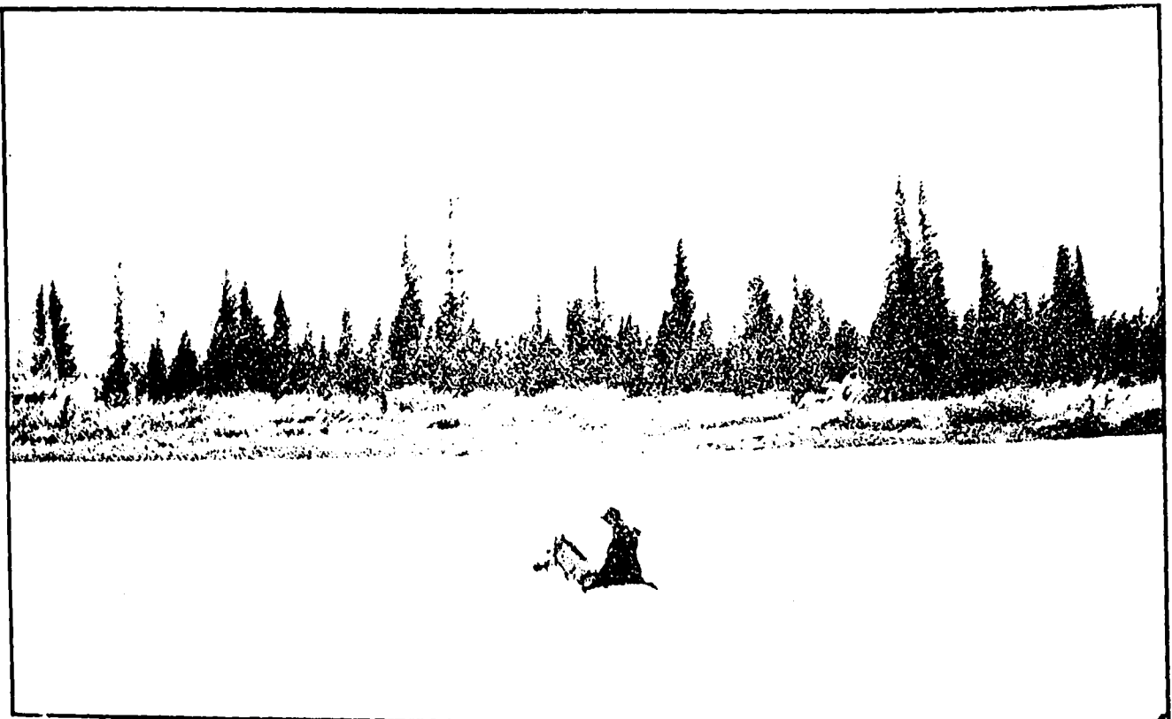
SWIMMING THE BOW RIVER. A BRIDGE WILL BE BUILT HERE AS PART OF THE NEW ROAD
