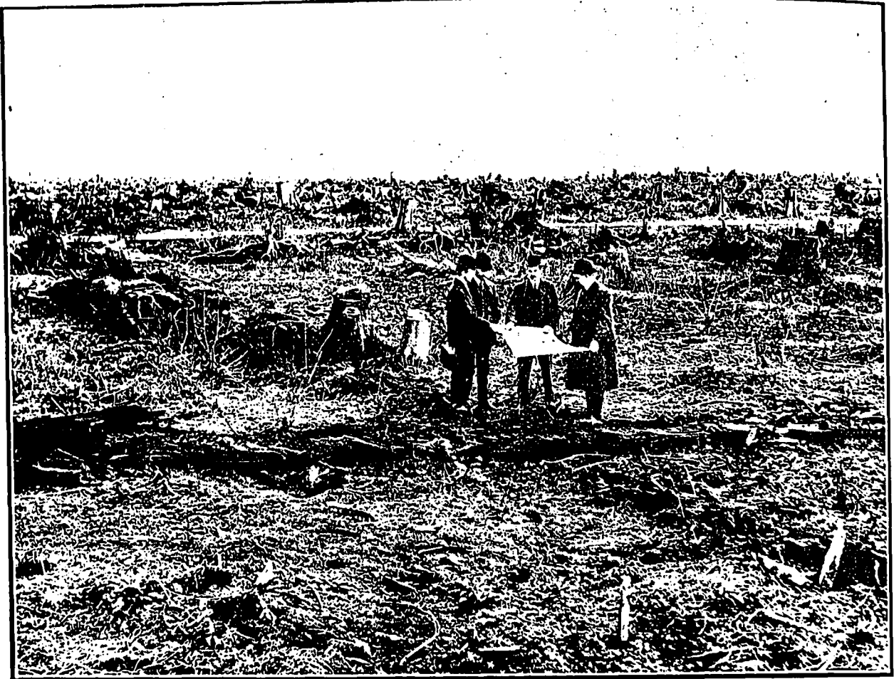
THE SITE OF MANLEY'S HOTEL AT PORT MANN. BUILDING OPERATIONS HAVE JUST COMMENCED ON THIS SPOT
