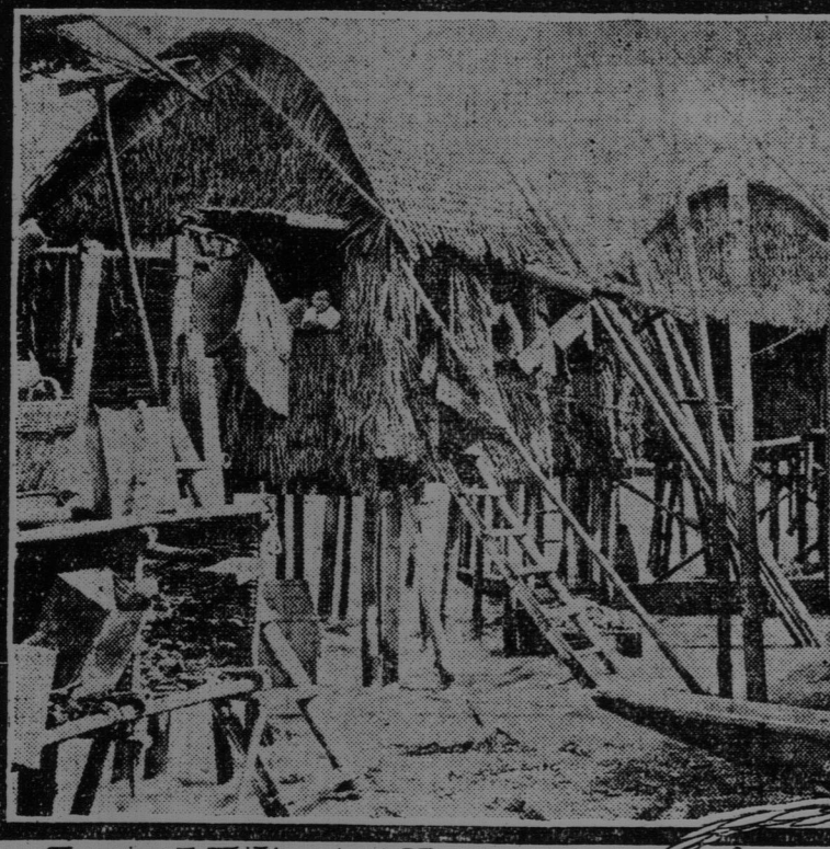
Typical Filipino Homes where the Plague Rages
