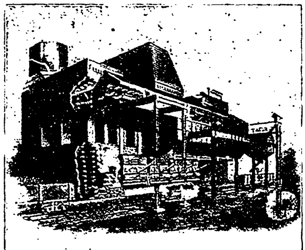
Storage Capacity 1,500 tons.
