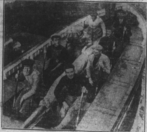
This new type of lifeboat which was recently tried out in England, is operated by moving levers to and fro, which operate a screw propeller. Some of the advantages of this type of vessel are that it can be got away from a ship's side in more or less awkward in manipulating oars at anytime let alone during a catastrophe at sea.
