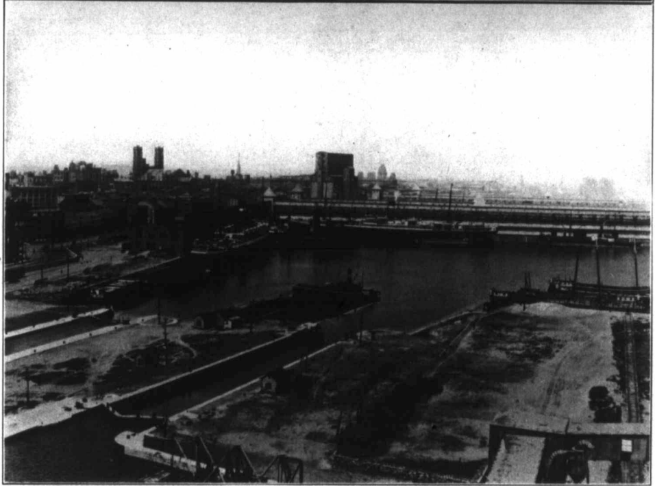
Port of Montreal—Elevator Building—The Reconstructed Harbor.
