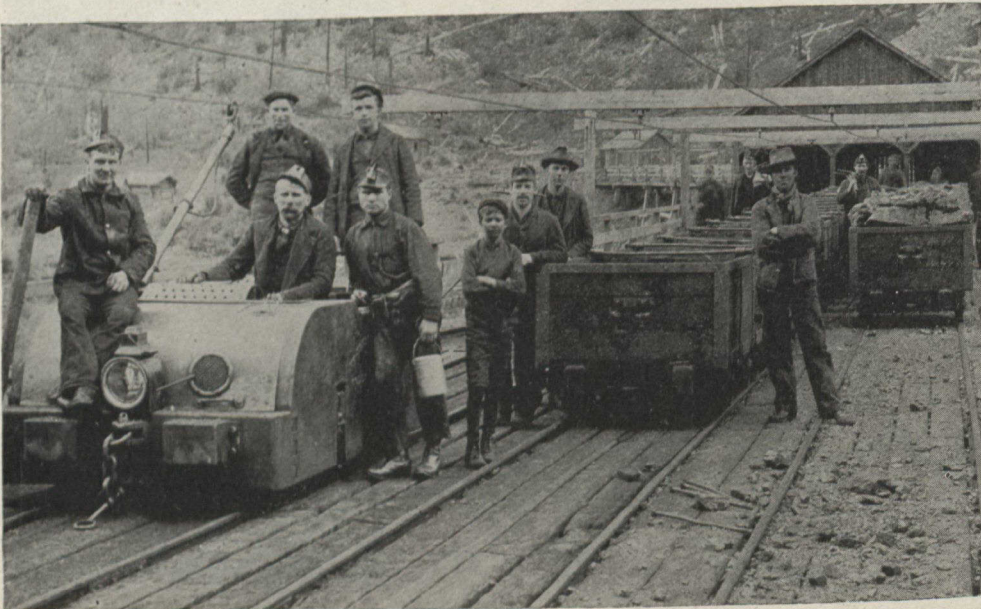
Mouth of one of Crow's Nest Coal Company's Coal Creek Mines, showing Electric Haulage Trolleys, Mine Cars, Drivers and Miners.
