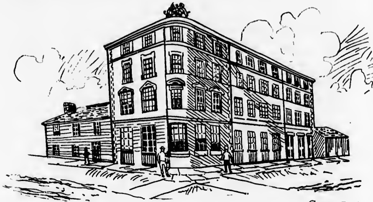
BUILDING, ON THE SOUTH-WEST CORNER OF CHURCH AND COLBORNE STS., WHERE KING SOLOMON'S LODGE MET, 1855-67.
