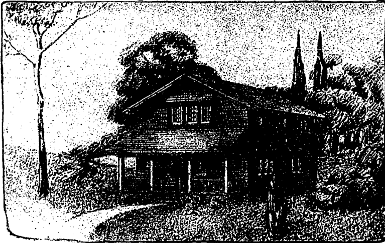
Design No. 5. A small house with shingle covered wall. The simplicity of its lines is relieved by the overhanging eaves and rafter, the well balanced porch, grouping of windows and heavy beams which extend around wall. This design will admit, in a limited way, of the substitution of other materials.
