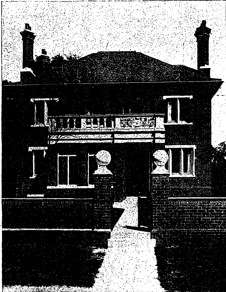
Front view, Residence of Mrs. W. P. R. Street, Toronto, showing brick garden wall and general detail of facade. W. A. Langton, Architect.
