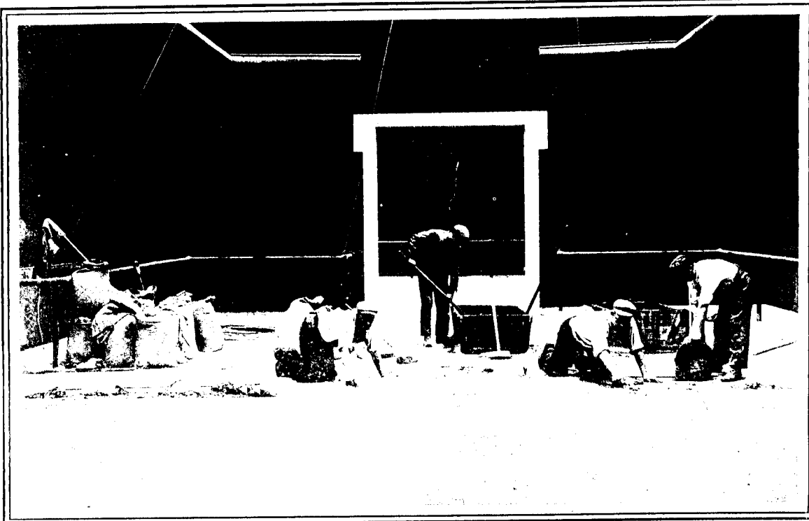
The above is a photograph of TERRANO FLOORING being laid in Art Gallery of Toronto Exhibition, seven hundred and seventy-five square yards. Prices and samples on application to
