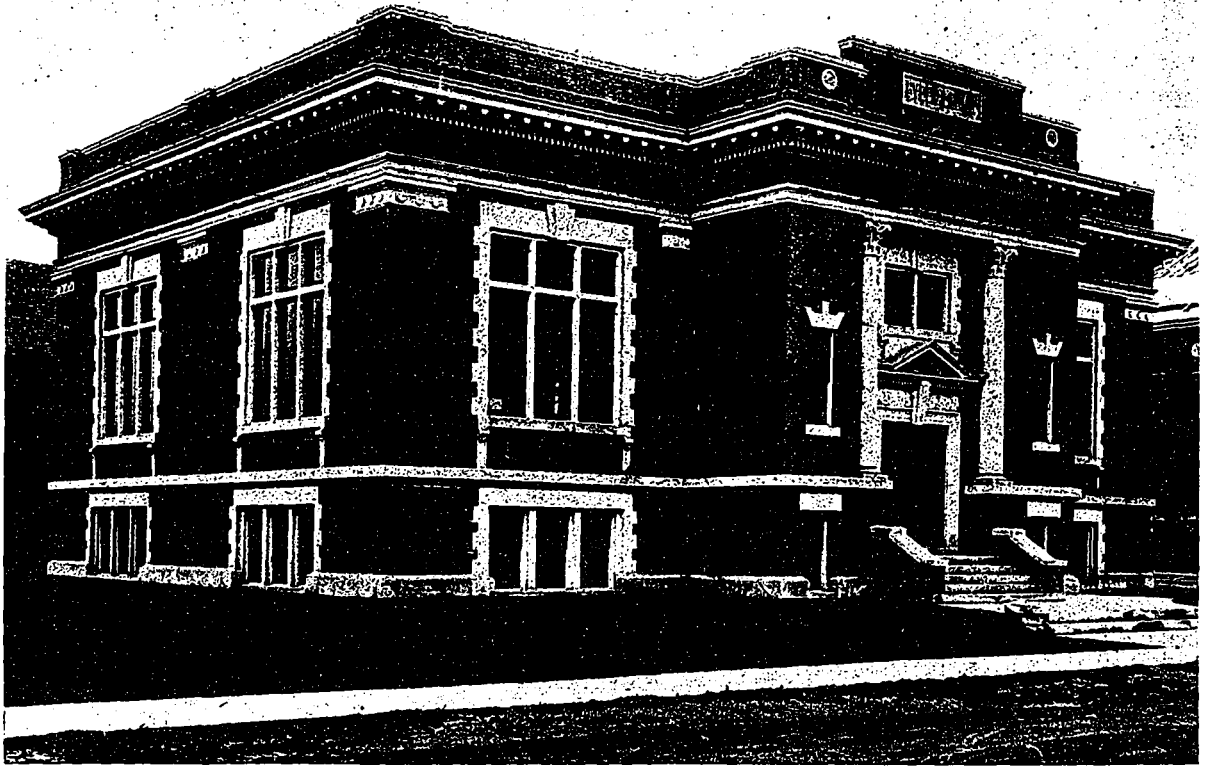
New Public Library, West Toronto. Ellis and Connery, Architects.
