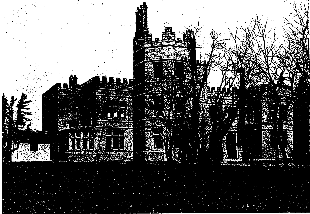
Residence of Mr. A. Ansley at "Glen Grove," an estate in Eglinton, a suburb of Toronto. Geo. W. Gouinlock, Architect.
