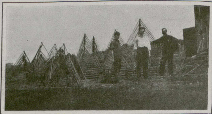
Tetrahedral Units from which the Tower was Built.
