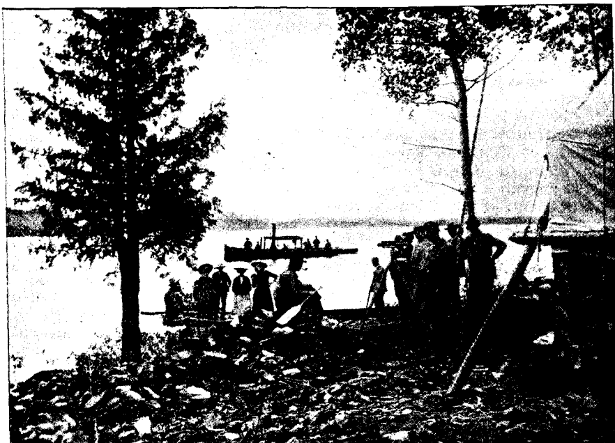
At the Engineer's camp.
