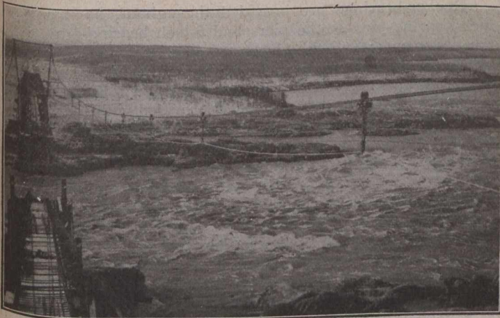
Fig. 7—View from Top of Cableway-tower
