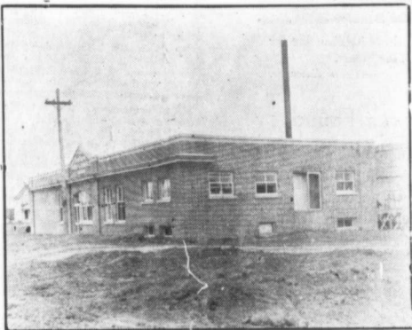
Substantial Evidence of Western Dairy Development
