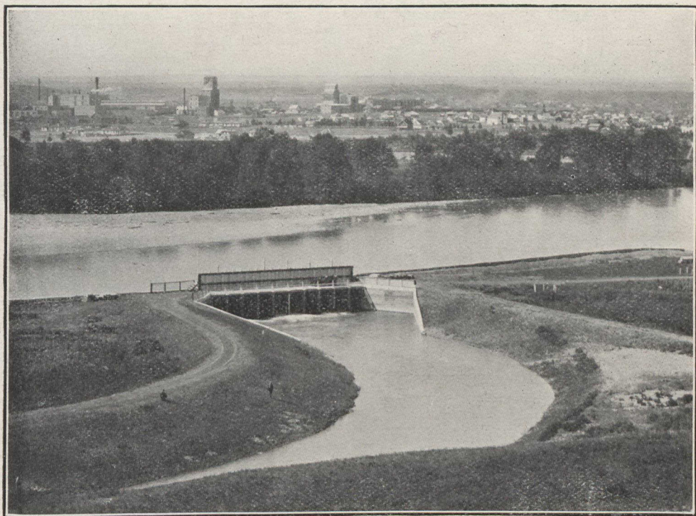
Headgates of the C.P.R. Irrigation Canal, Calgary, Alta.
