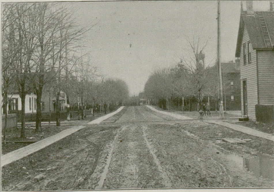
WHERE GOOD AND BAD ROADS MEET.
