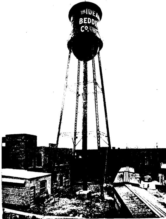
Steel Water Tank and Tower, Ideal Bedding Co., Toronto. Coated with Bitunamel.
