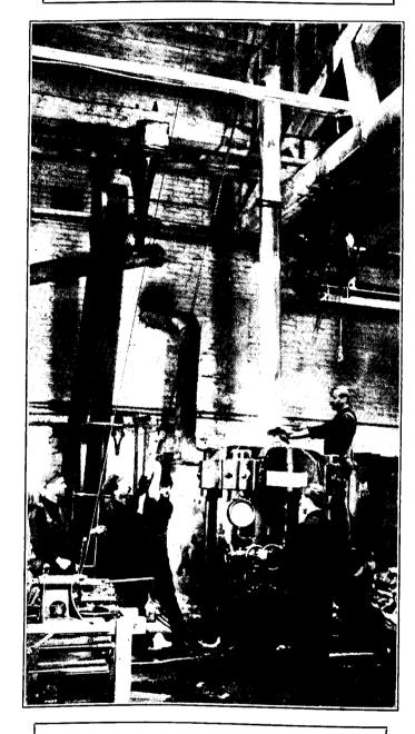
This illustration shows a length of 8 inch lead pipe, weighing over 500 lbs. being taken from the press.
