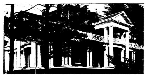
The above verandah contains 8 columns, 24 in. diameter x 20 ft., and 23 columns 12 in. x 10 ft., which were manufactured by us.
