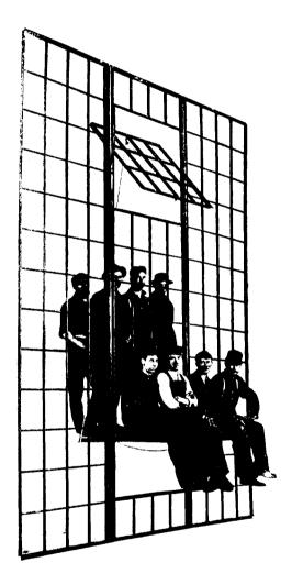
The muntins are deep and narrow, offering a minimum obstruction to the light. The joints are not weakened in any way by cutting or punching.
