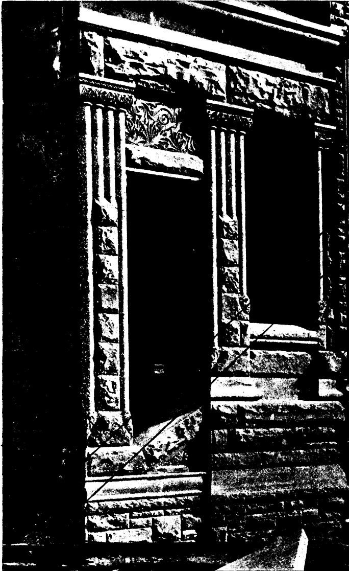
PRIVATE ENTRANCE, NORTH-EAST CORNER.
