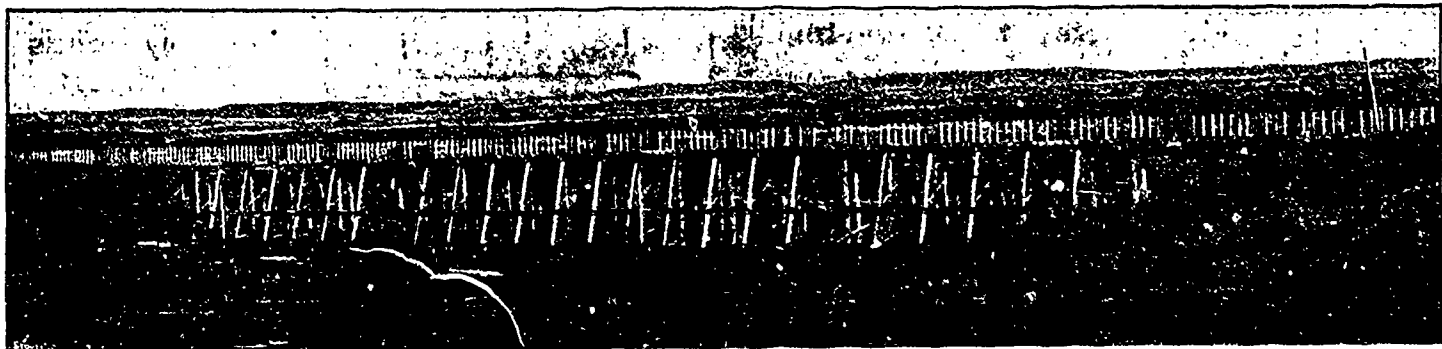
Flume, 784 Feet Long, with Trestles 28 feet high, carrying canal over bed of Willow Creek
