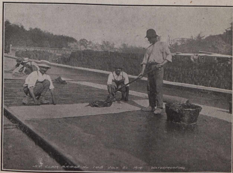
Fig. 12.—Illustrating the Three Stages of Waterproofing.
