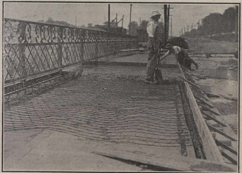
Fig. 11.—Method of Reinforcing Sidewalk Slab.
