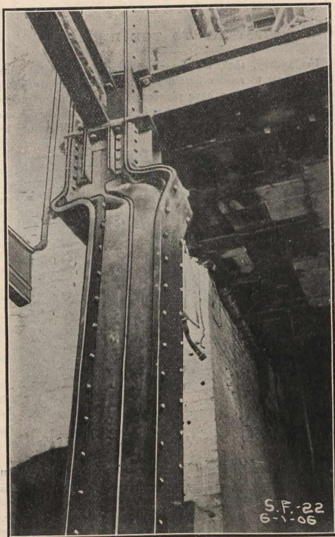
Earthquake Effect on a Steel Beam: Unprotected.
