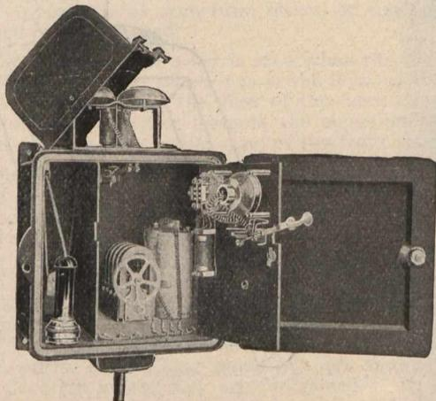
Fig. 2.—The Mine-A-Phone: Open View.
