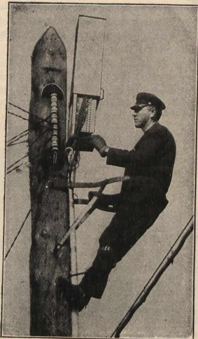
The Robinson Distribution Rack, Especially Useful for Taking Off Leads Running from Only One Side of the Pole.
