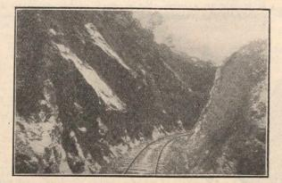
Fig. 5.-Example of Rock Cutting.
