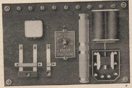
Fig. 4.-Test Switch-Board.
