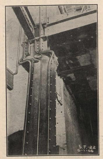
Earthquake Effect on a Steel Beam: Unprotected.
