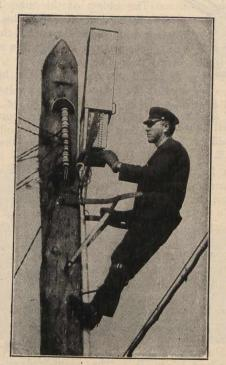
The Robinson Distribution Rack, Especially Useful for Taking Off Leads Running from Only One Side of the Pole.
