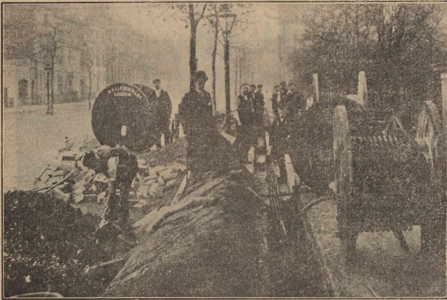
Laying Callender Mains at DONCASTER.
