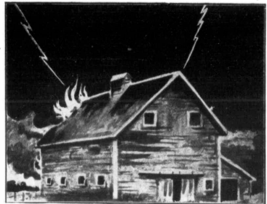
UNPROTECTED—Ruined in a Moment.
