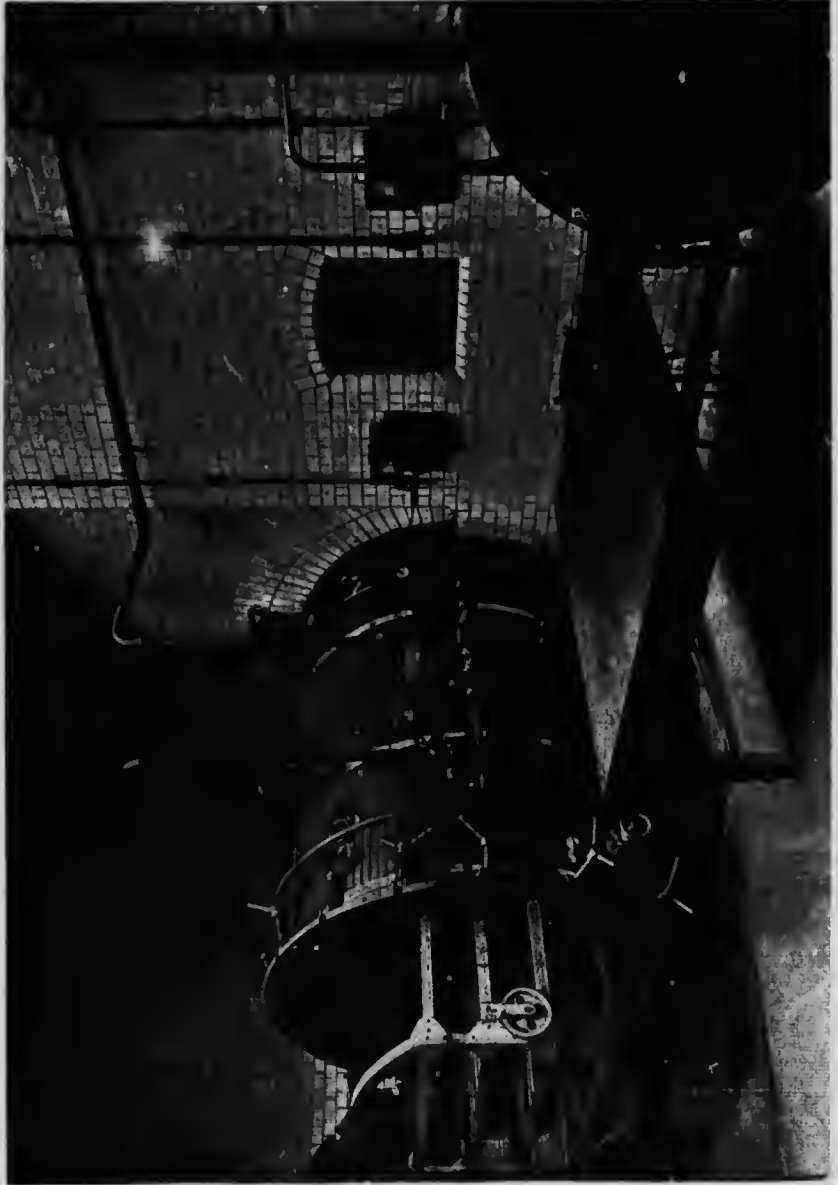
FIG. 90.—(c) DISINFECTING STATION. INFECTED SIDE.
