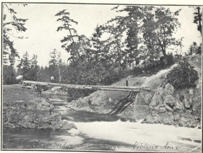
FIRST BRIDGE OVER THE GORGE, VICTORIA ARM.
