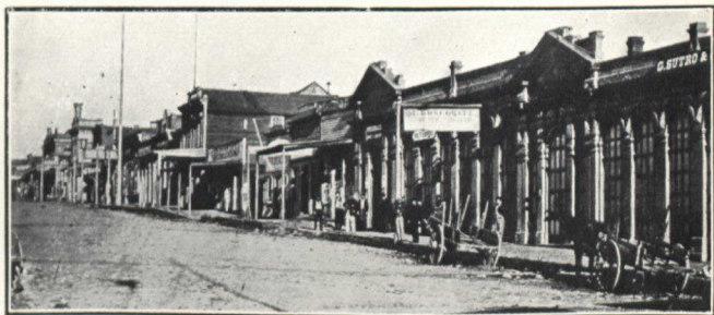
YATES STREET, LOOKING EAST.
