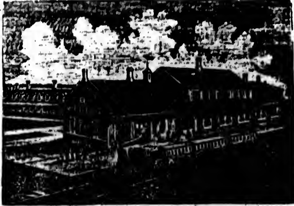
GRAND TRUNK RAILWAY PASSENGER STATION.
