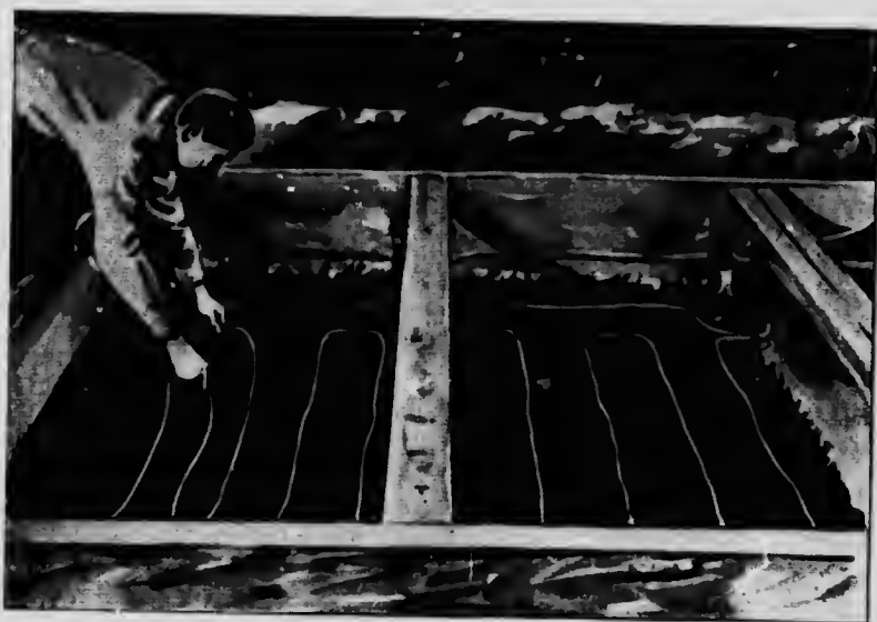
Preparing the electric hotbed, showing how the heating cable is laid.
