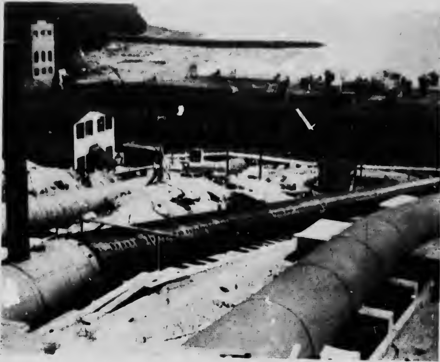
Powell River Development. General view of Pipe Lines.
