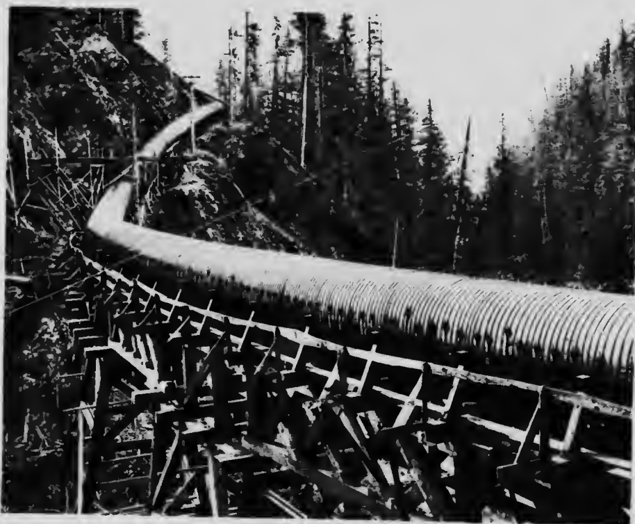
Granby Consolidated Mining, Smelting and Power Company Limited. 72 Inch Wood Stave Pipe Line on Trestle.
