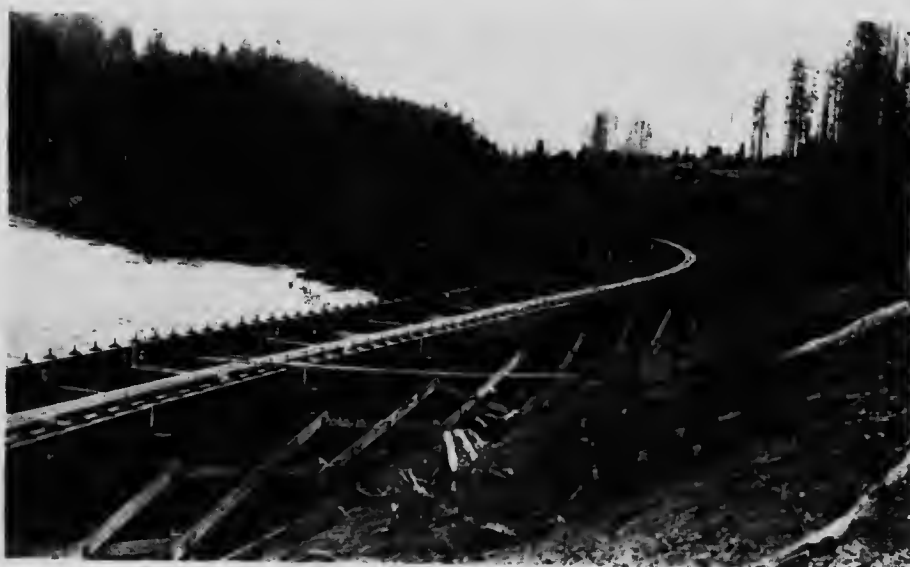
Canadian Collieries (Dunsmuir) Ltd. General view of Flume.
