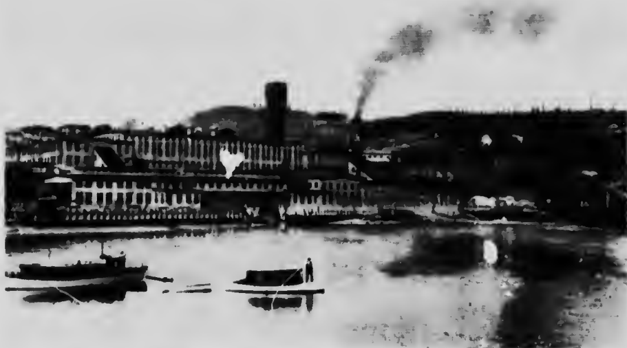
Powell River Development. General view of the Paper Mill (taken before date of inspection).
