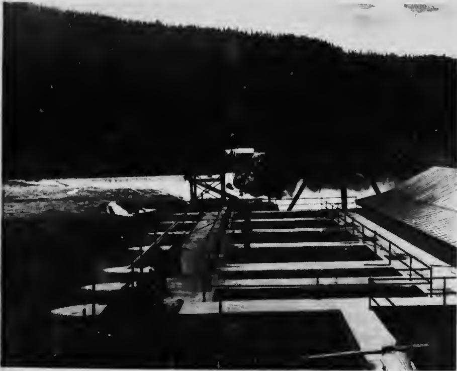
Kootenay River Development. Head Works, No. 2 Power House. Upper Bonnington Falls.
