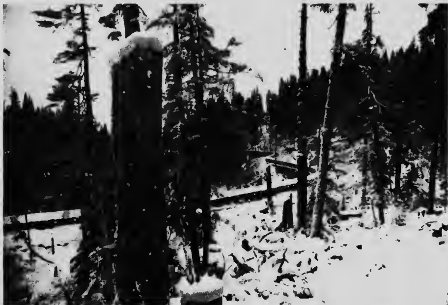
Granby Consolidated Mining, Smelting and Power Company Limited. 72 Inch Wood Stave Pipe Line under Winter conditions.
