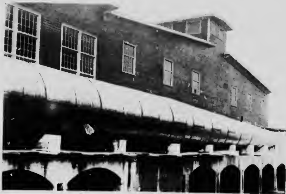
Ocean Falls Company Limited. Pipe line at back of Power House.
