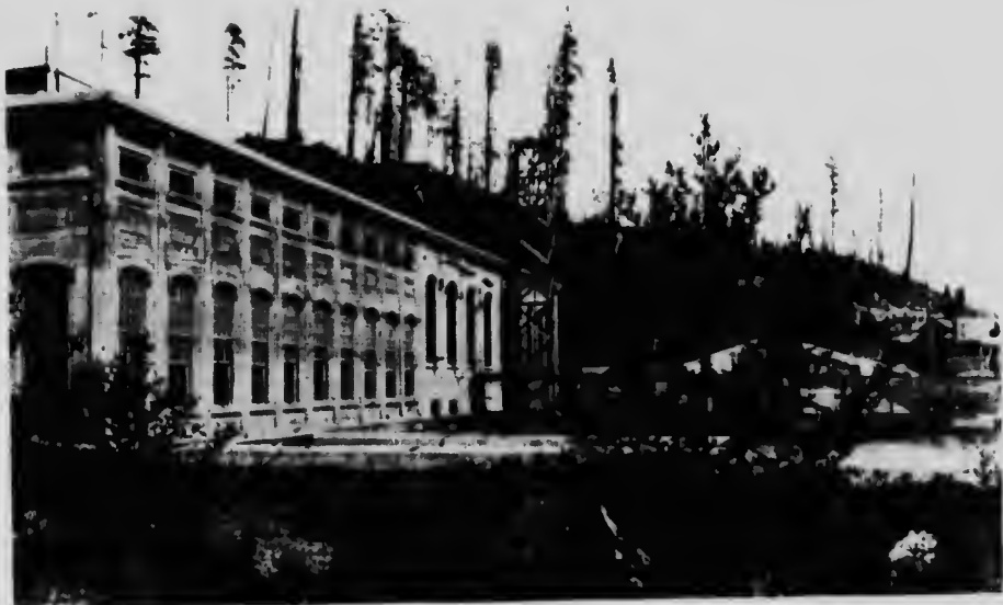
Vancouver Island Power Company Limited. Looking East, showing front of Jordan River Power House.
