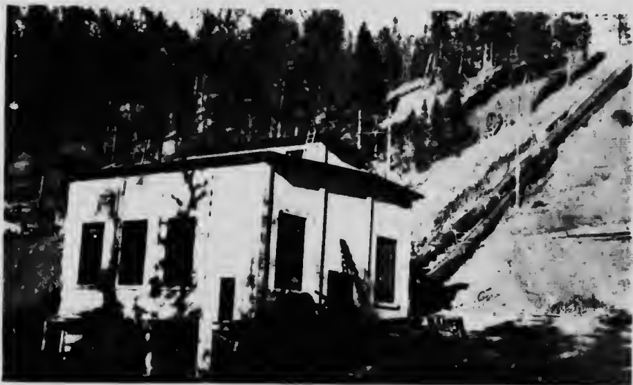
City of Kamloops-Barriere River near Kamloops. Barriere Hydro-Electric Generating Station.
