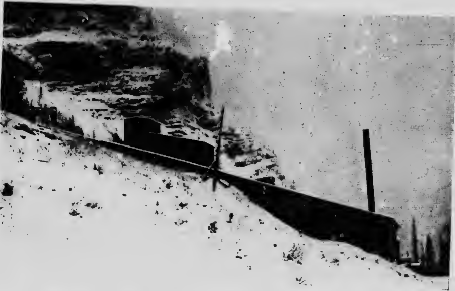
Cathedral Creek Development. Concentration Plant and Power House, Mount Steven Mine.
