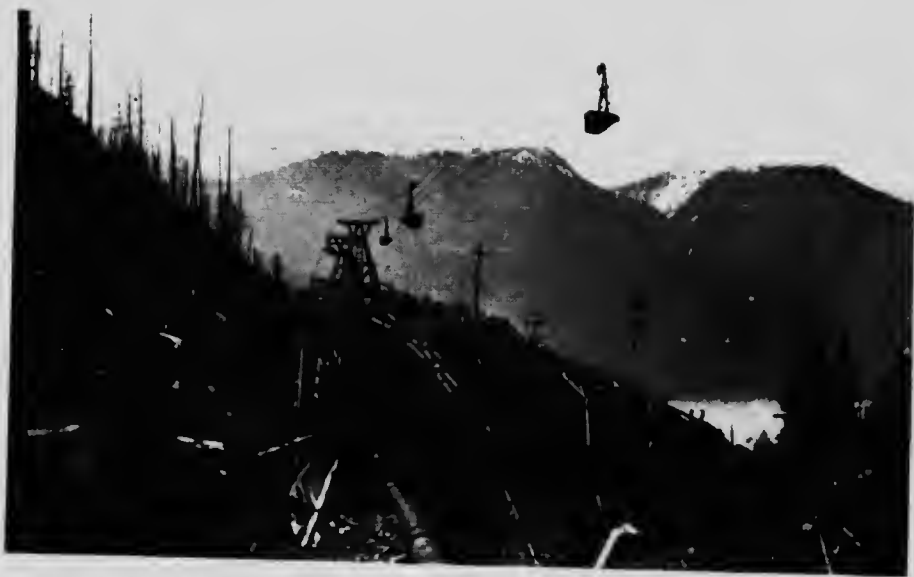
Britannia Mining and Smelting Company Limited. Aerial Tramway conveying Ore from Britannia Mine to the Mills at Britannia Beach. Howe Sound is seen on the right of the picture.
