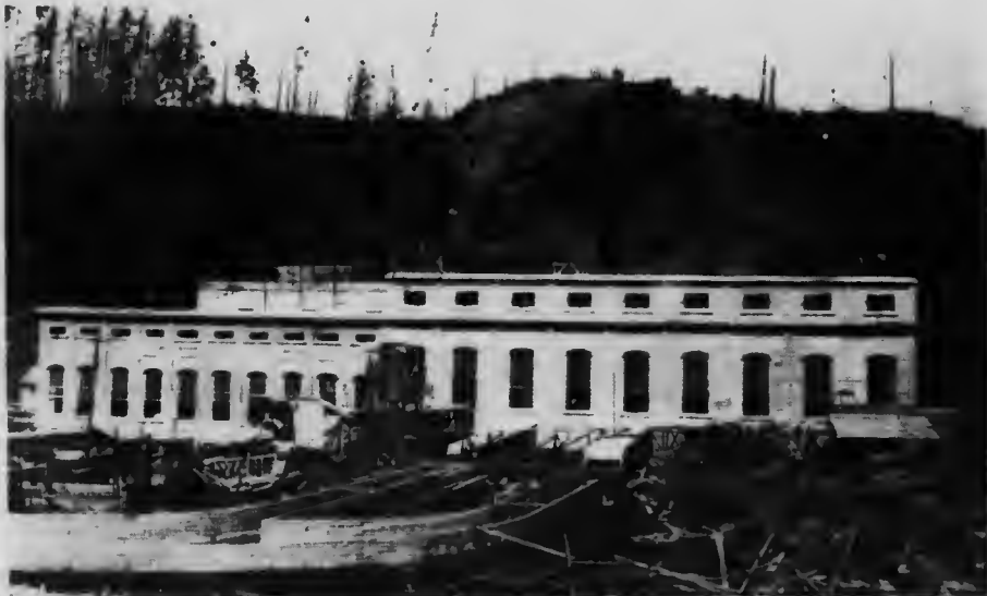
Vancouver Island Power Company Limited. Front view of Power House showing completed building and tailraces.
