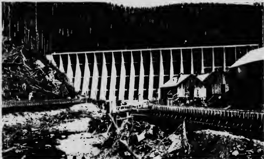
Vancouver Island Power Company Limited. Downstream face, Jordan River Dam.
