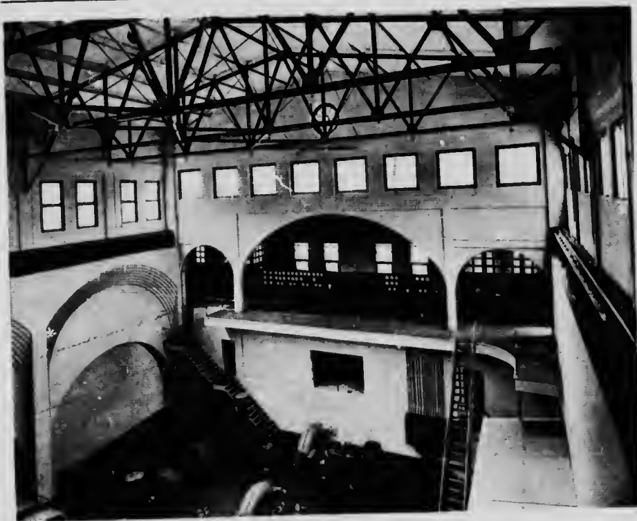
Stave Falls Development. Switchboard, Stave Falls Power House.
