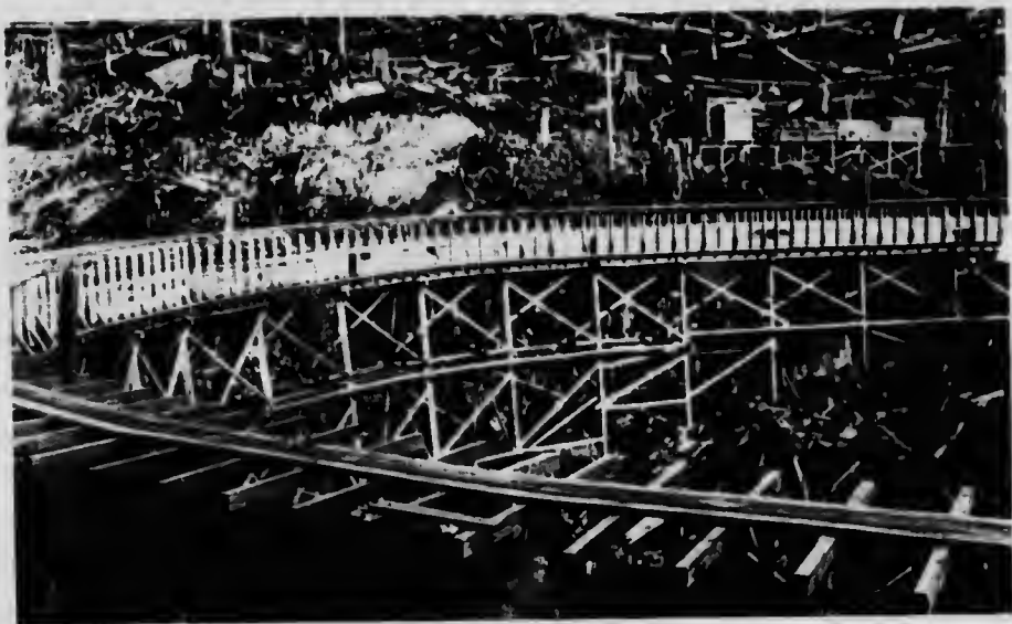
Vancouver Island Power Company Limited. Flume between Jordan River Dam and Forebay Reservoir.
