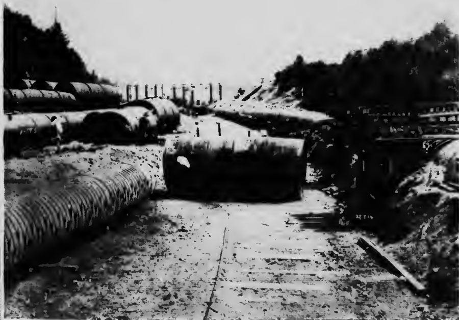
Coquillam-Buntzen Development. Replacing wood stave pipe lines with rivetted steel pipes.
