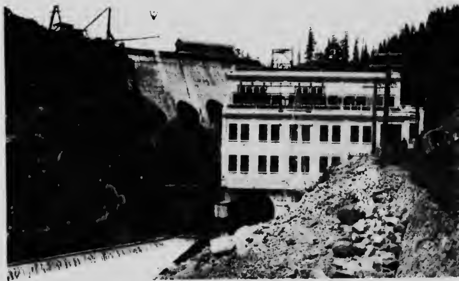
Stave Lake Development. Stave Falls Power House.
