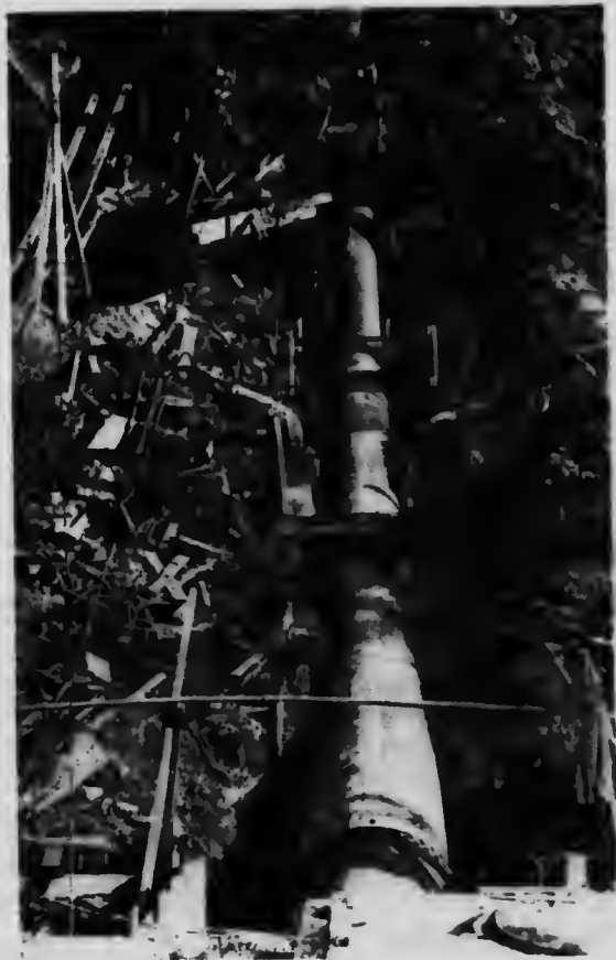
Vancouver Island Power Company Limited. No. 3 Pipe Line as seen from Power House.
