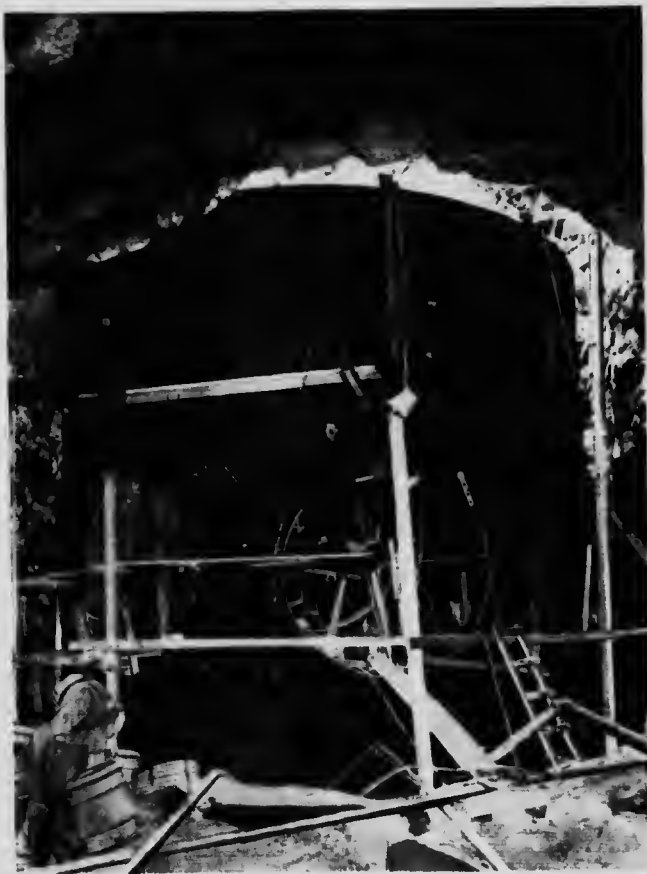
Coquitlam-Bunzen Development. Surge tank, showing openings for pipe line connections.
