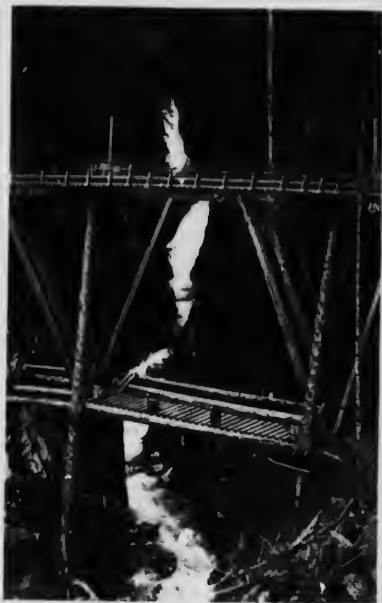
Britannia Mining and Smelting Company Limited. Bridge carrying Electric Railway over Britannia Creek.
