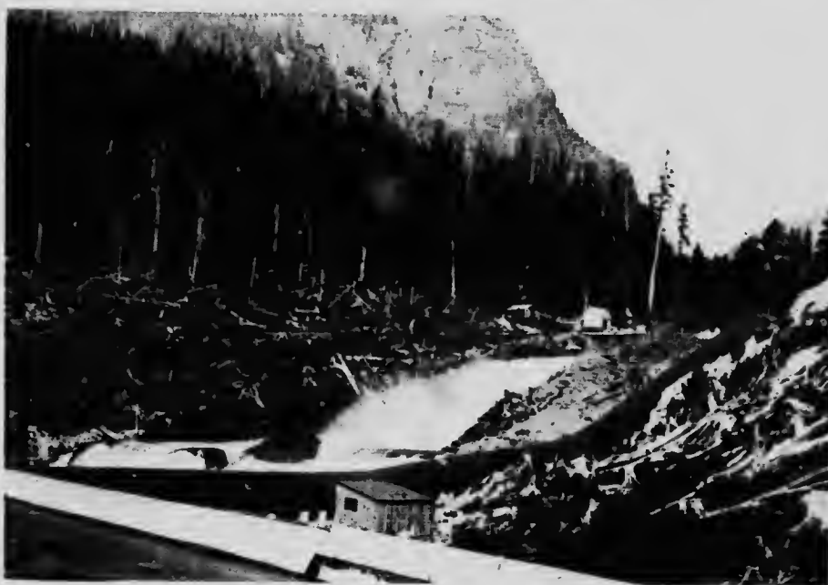
Ocean Falls Company Limited. Pipe line and Link River near Power House.
