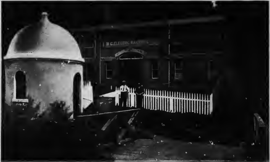
British Columbia Electric Railway Company, Limited. Goldstream Power House.
