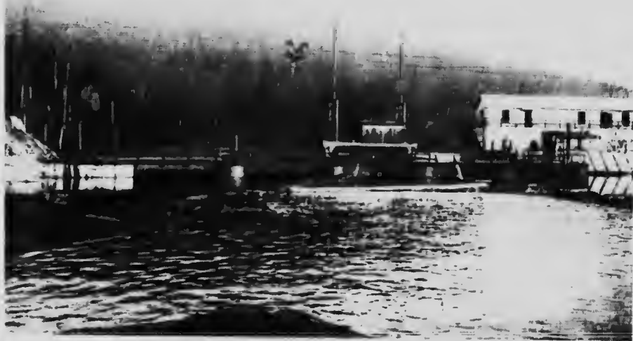
Stave Lake Development. Looking downstream above dam.
