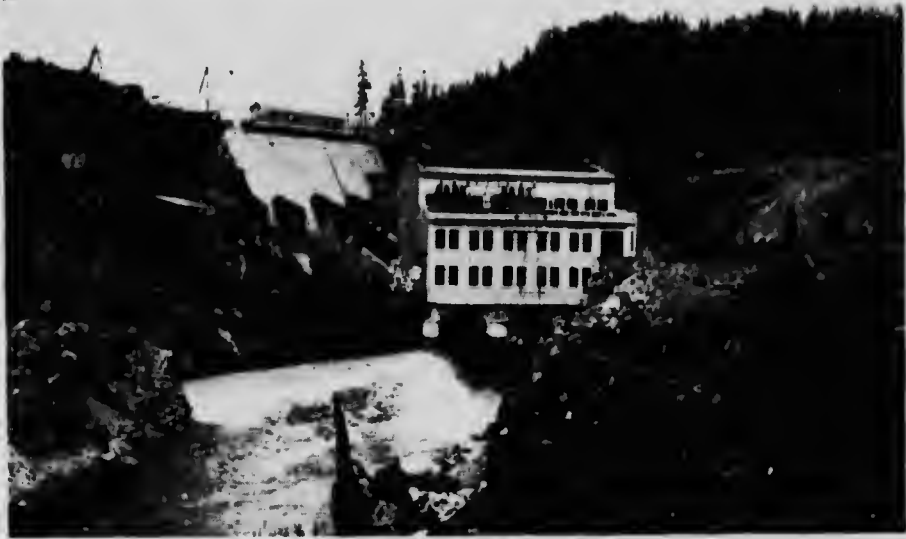
Stave Lake Development. Power House, Stave Lake.
