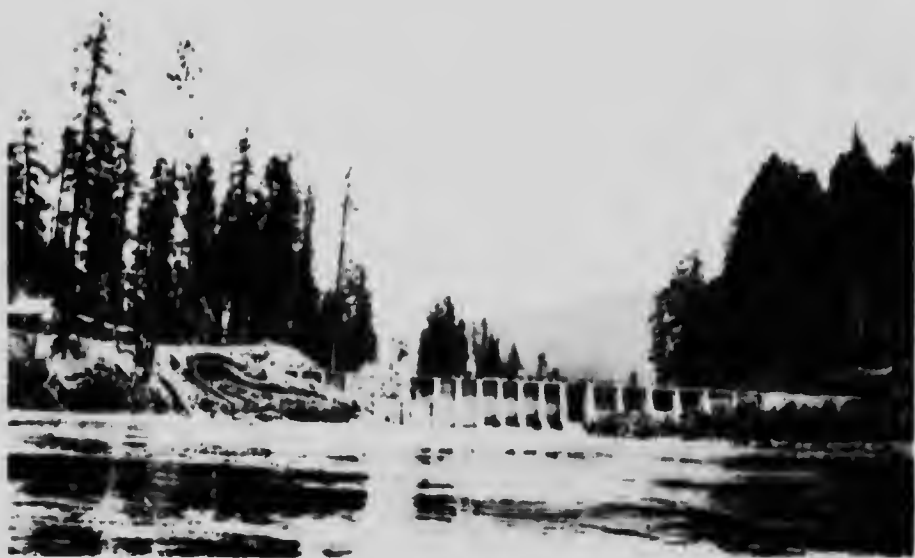
Canadian Collieries (Dunsmuir) Ltd. Storage Dam.
