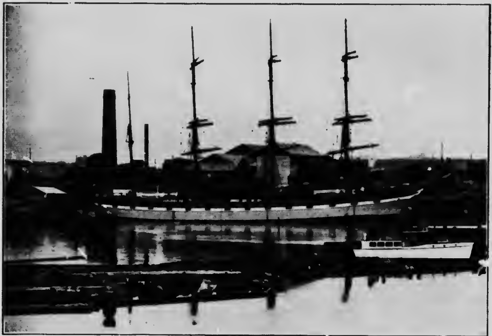
"Kinross-shire," Loading about 2,000,000 feet of Lumber Canadian Puget Sound Lumber Co.'s Docks, Inner Harbor
