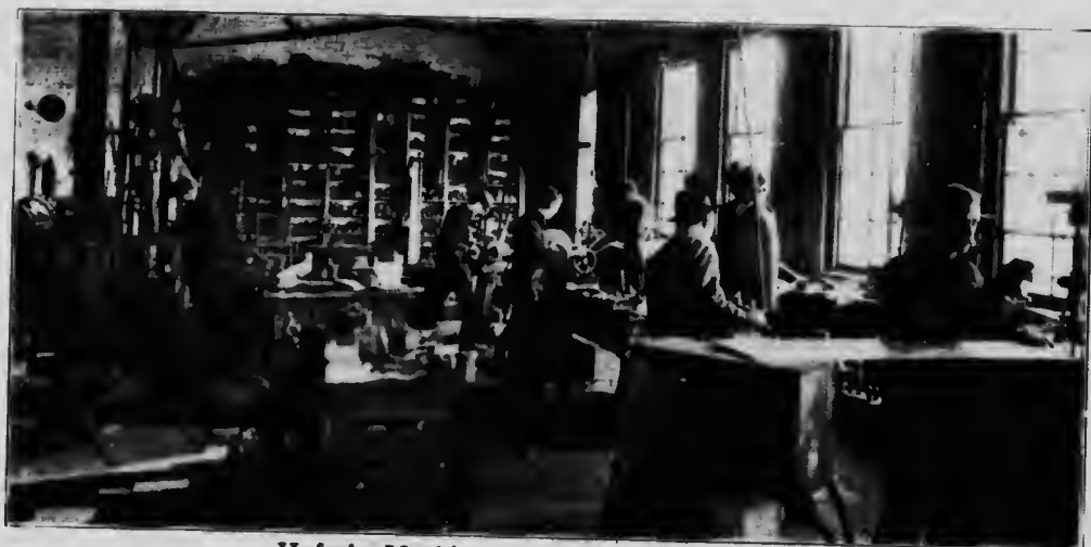
Hafer's Machine Works—Finishing Room
