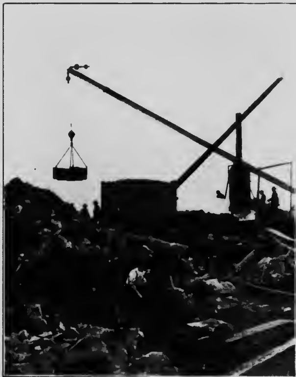
At Work on Outer Harbor Additions, Victoria, B. C.
