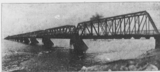
Victoria Jubilee Bridge, Montreal, P.Q. Intercolonial Route.
