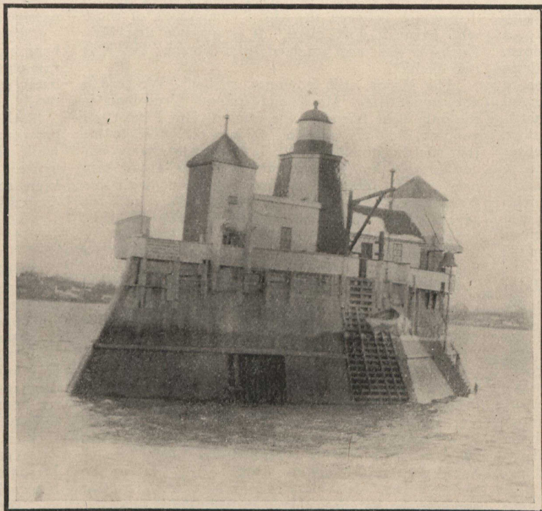
Beacon Light in St. John Harbour, the pier is of cribwork and has been repeatedly repaired.
