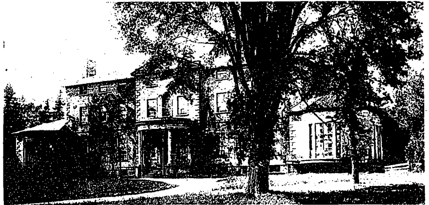
HUNDRED YEAR OLD GOVERNMENT HOUSE, FREDERICTON, N.B., BEING RECONSTRUCTED AND ADDED TO AS A CONVALESCENT HOSPITAL.
