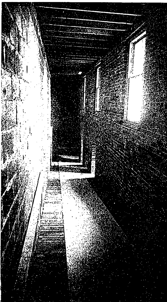
UPPER SECTION OF RUNWAY AT CAMP HILL HOSPITAL.
