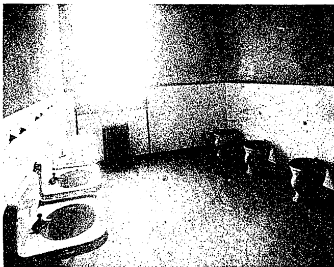
ONE OF THE TOILET ROOMS IN CAMP HILL HOSPITAL BEFORE CLOSET PARTITIONS WERE ERECTED.
