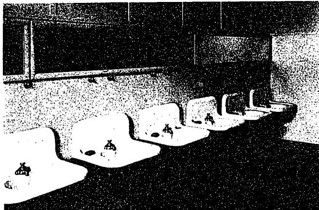
WASH ROOM AT MANITOBA MILITARY HOSPITAL.
