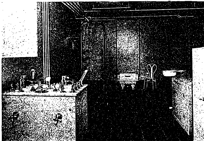
TREATMENT ROOM AT COBOURG, SHOWING NOZZLE, NEEDLE AND CABINET BATHS.
