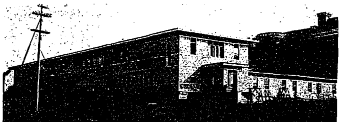
JULY 25—EXTERIOR COMPLETED AND SCAFFOLDING DOWN.
