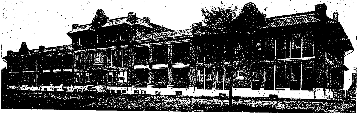
MAIN BUILDING OF MOUNTAIN SANATORIUM, HAMILTON, ERECTED BY HAMILTON HEALTH ASSOCIATION AND TAKEN OVER BY MILITARY HOSPITALS COMMISSION.
