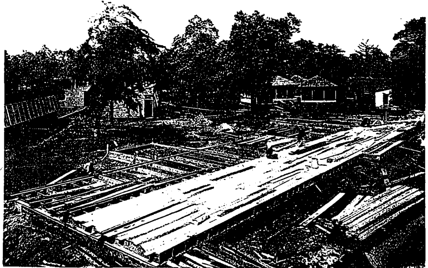
BEGINNING CONSTRUCTION OF LARGE NEW PAVILION AT MOWAT SANATORIUM, SHOWING SEVERAL JUNIOR PAVILIONS IN BACKGROUND.
