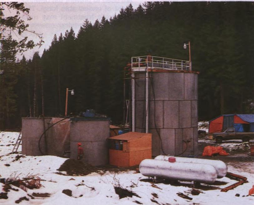
The largest biological leaching reactor in the world. The tank measures 6.5 m in diameter and 7.2 m in height. This reactor is located near Goldbridge in British Columbia.
