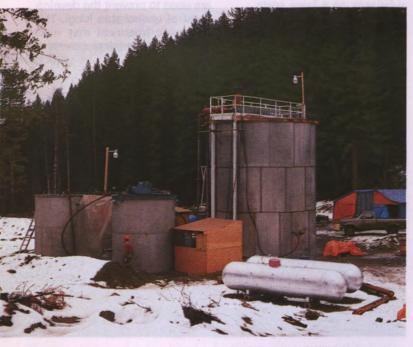
The largest biological leaching reactor in the world. The tank measures 6.5 m in diameter and 7.2 m in height. This reactor is located near Goldbridge in British Columbia. (GB Biotech Inc.)
