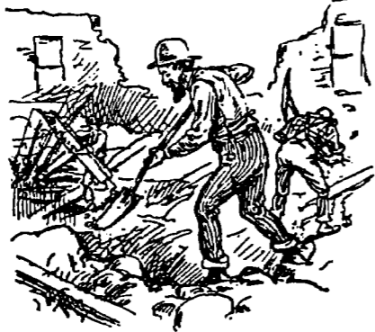
"I was helping dig out the cellar."
