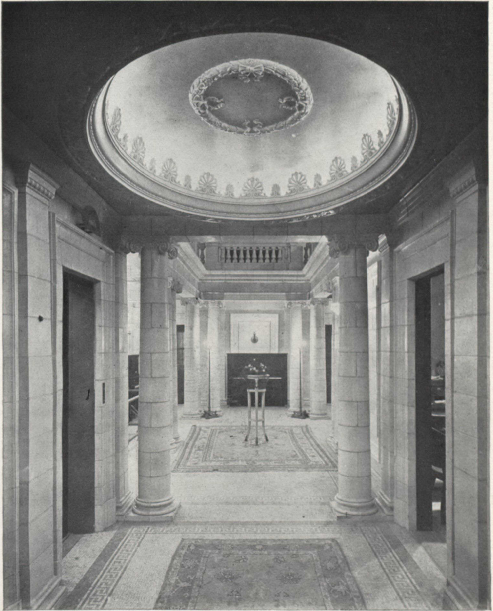
LOOKING INTO THE ROMAN COURT, MASON & RISCH BUILDING
