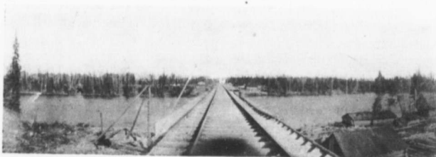
VIEW OF MATTAGAMI RIVER, LOOKING EAST—FIRE RANGERS' CAMP MARKED IN WOODS.
