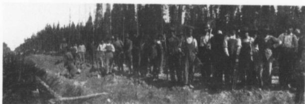
LIFT GANG ON CONSTRUCTION.
