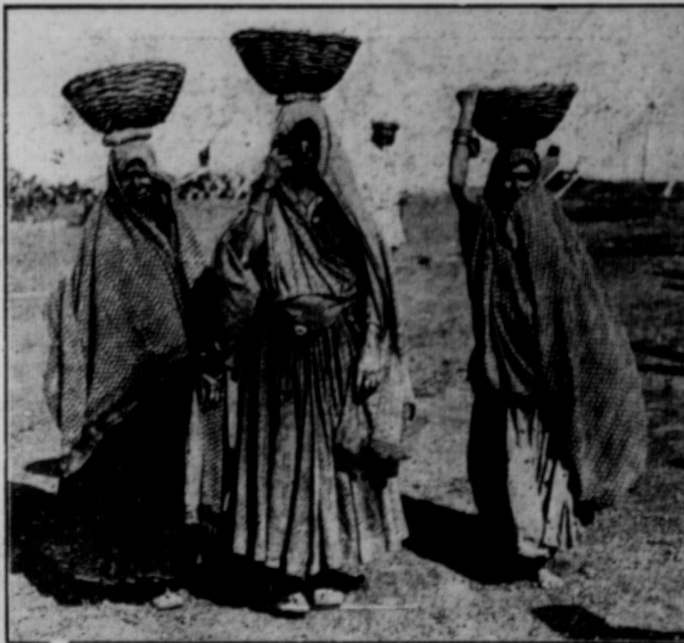
NATIVE WOMEN IN INDIA CARRYING STONE FOR ROAD-MAKING
