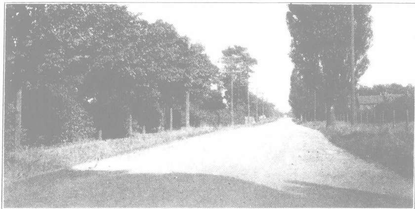
Danforth Road, York County Highway Board, Ontario. Treated with "Tarvia-B" in 1916.
