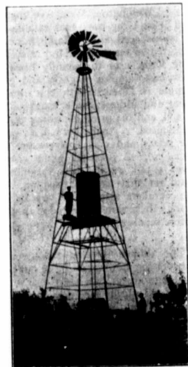
Brantford Steel Windmill and Tower in Russia.
